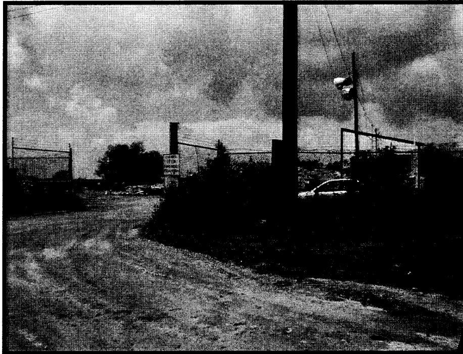
Entrance to the demolition debris/transfer station at the former landfill.
